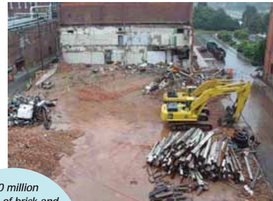
Former location of Building 2 showing the segregation of building materials to facilitate recycling and reuse.
